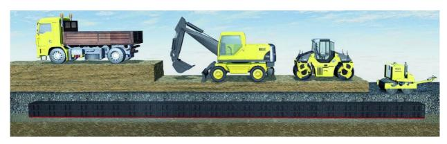
Various construction machinery may be used to fill the excavation. Given the additional dynamic loads they cause, compression equipment must not be driven directly over the RAINBOX CUBE system and compression equipment with activated vibration motors must not be taken over the area.
