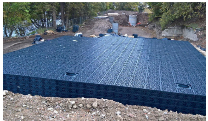
Housing Estate, Aberdeenshire (UK)
